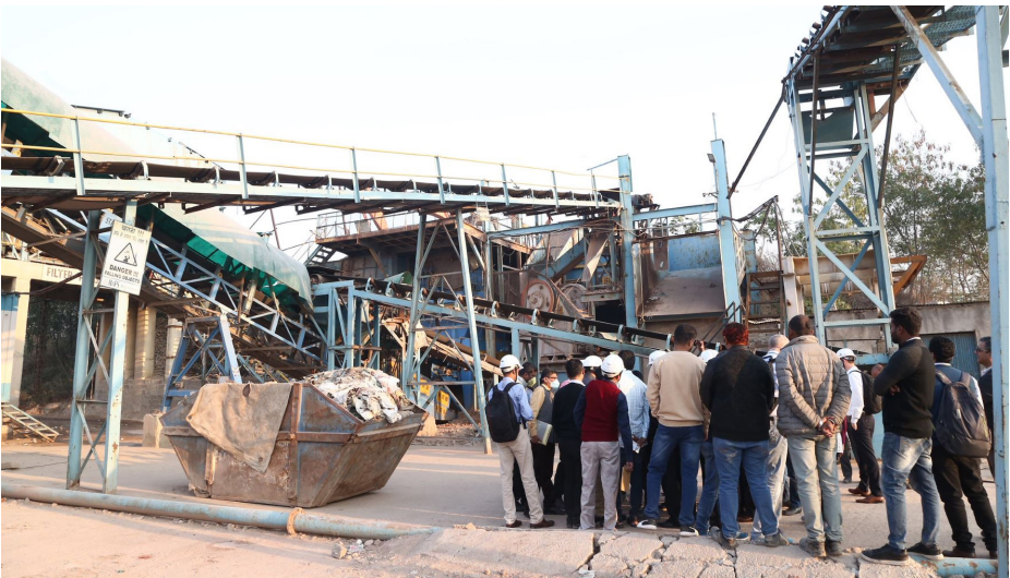
Figure 13: Visit of Burari Processing Site, Delhi
