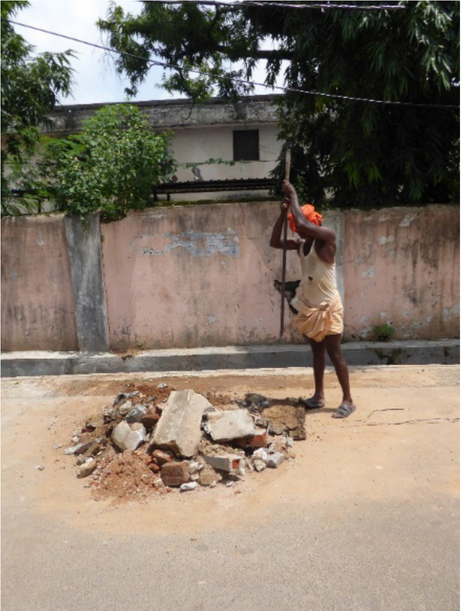
Figure 8: CDW Waste Recycling, separating concrete and bricks from concrete reinforcements
