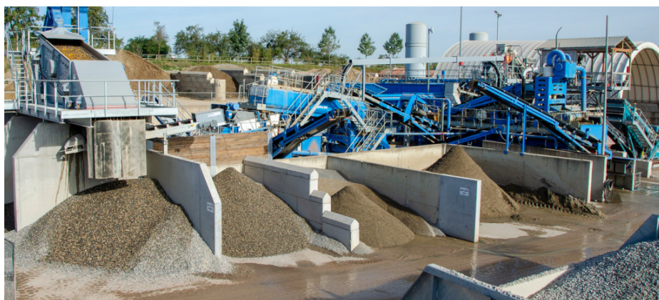
Figure 20: Wet classification plant, RC-parc Kirchheim
